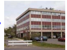
Office Buildings, Office Parks
